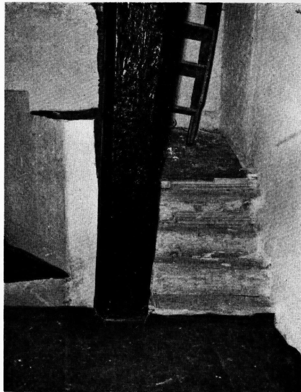
FIG. 12. The landing of the sixteenth-century stair showing spere post.
