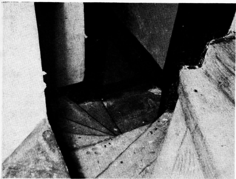
FIG. 19. The sixteenth-century stair.
