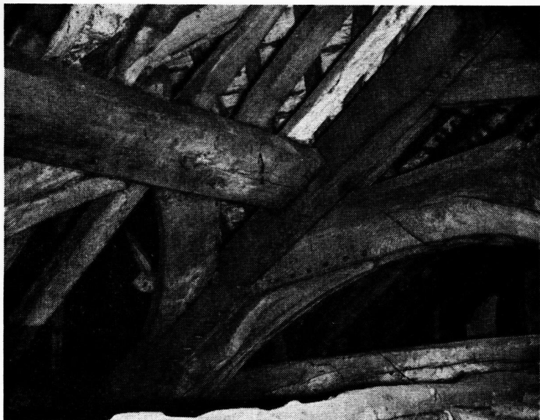
FIG. 13. The central truss, showing later cambered beam supporting ceiling.
